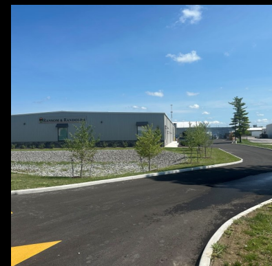
Completing R&R's 50% Expansion Maumee, OH production facility
